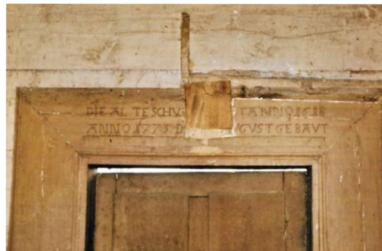
Lintel with inscription in 1978. Part of the inscription was damaged by the placement of a cross-beam sometime in the past.
